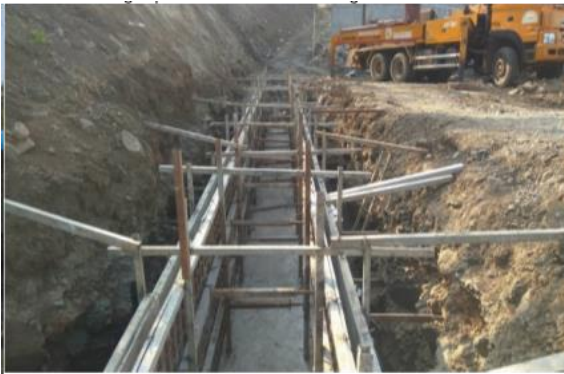
Feb 18: Drainage culvert construction STP
