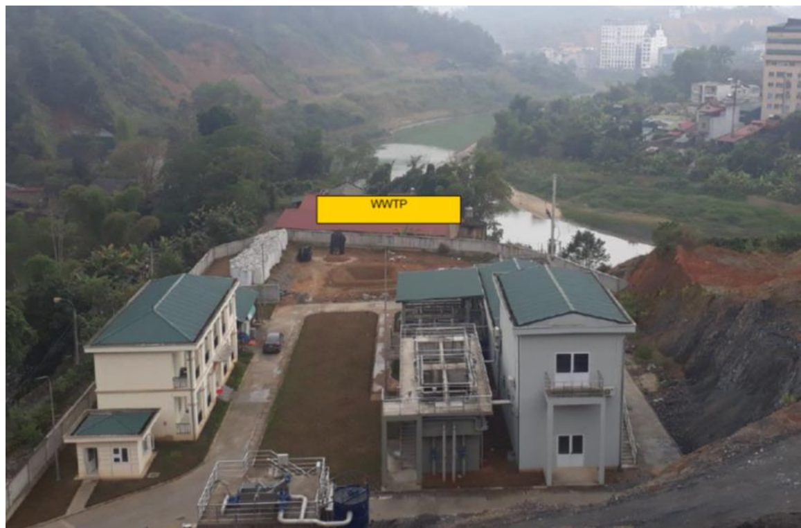
April 2021 Field Visit Project Photographs
