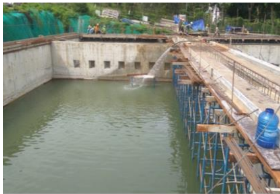
Sep 17: Leak testing of MBBR reservoir
