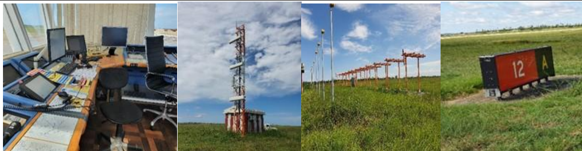
From left to right: Control tower equipment, traffic control, alignment / localizer and signalization.
