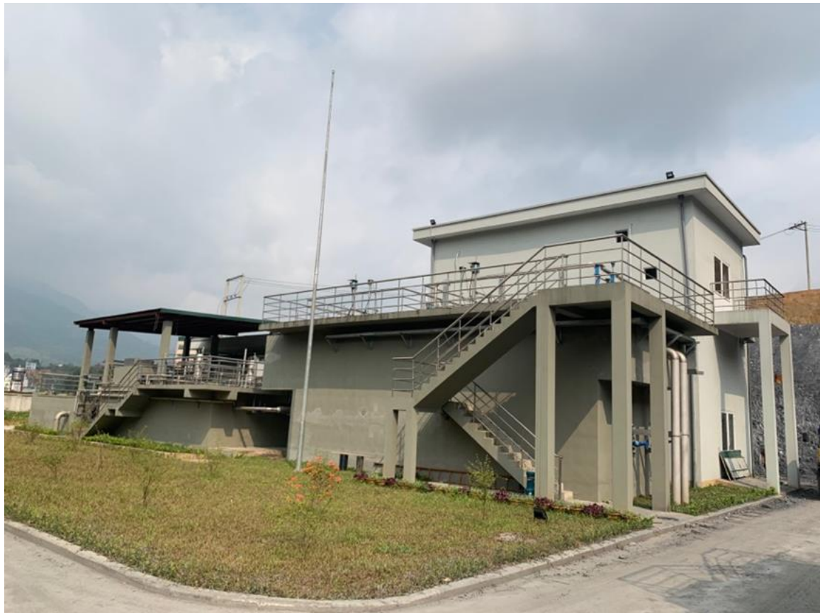
Wastewater treatment plant, April 2021
