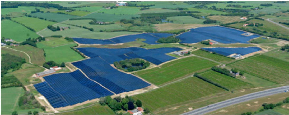
The world's largest solar heating plant on the outskirts of Silkeborg optimises the whole DH system. The green area between the two sections has been left untouched in order to make room for the future construction of a highway.
